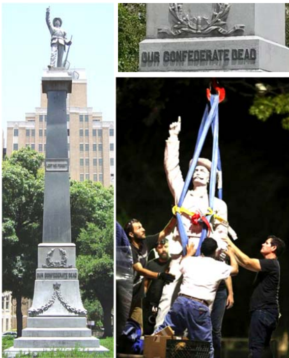
Left: Memorial before it was removed; top right: Wording on the memorial; Bottom right: Work Crew removes Confederate soldier from monument (San Antonio Express-News)
