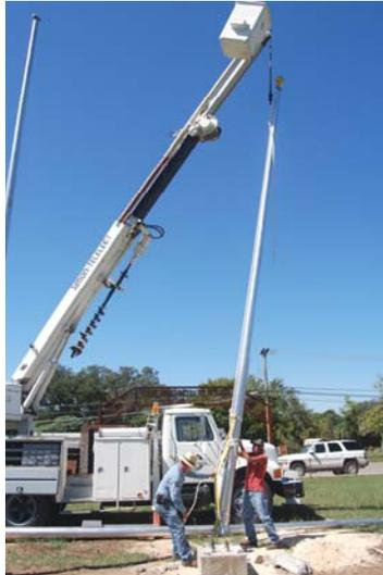
*Crane hoists new pole up as Rocky Sprott and James Kinnear line it in position.*
